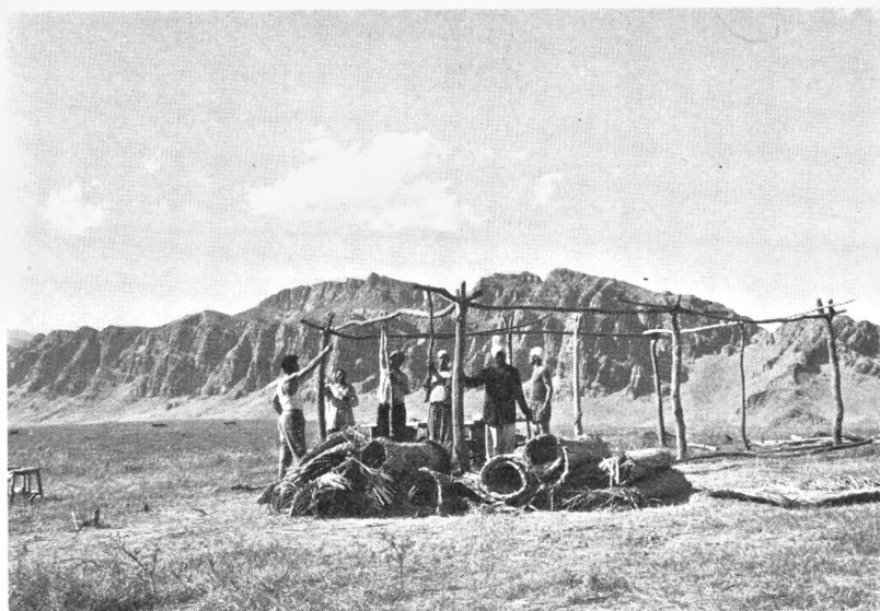
Fig. 7. Building of kapra on top of Camp Hill. May 1957.
